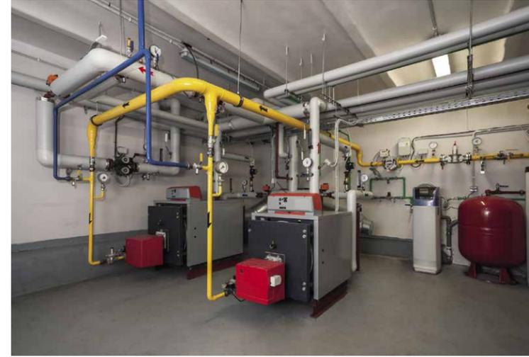
Figure 126: Condensing gas boiler
